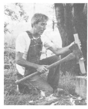
PLATE 131 Next, he drives the pegs into place in one of the two slabs. *Note:* In later steps, when the buckets are being cut out, these pins will be cut into. By that time, however, the two slabs will be held together by two iron hoops.
