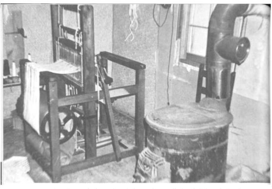
PLATE 299 Minnie Buchanan's loom, thrums all threaded through the dent and in place, waiting for a warp to be tied on.
