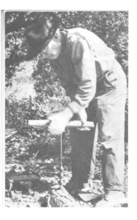
PLATE 65 Roughing out the yoke is a fairly simple process. After the size of the yoke to be made is determined (see diagrams), the sides of a piece of round stock of appropriate size are hewn off leaving a rough-hewn, rectangular block of wood. The outline of the yoke is drawn on the sides using a pattern—if one is available— or measurements. Then, with an auger, the four holes for the bows are drilled from the top surface in the proper places.
