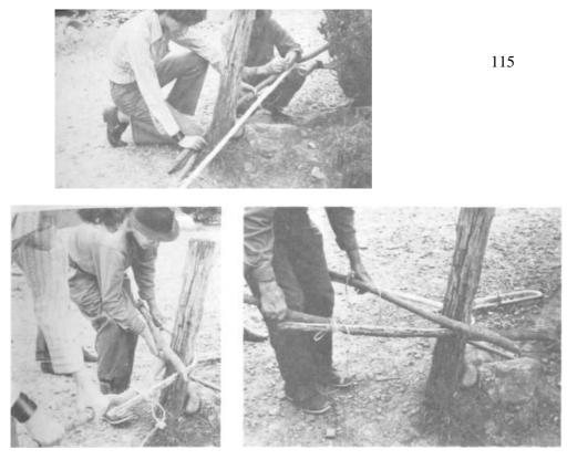
PLATES 67-69 With the yoke hewn out, the next step is to make the bows.
