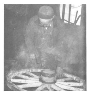
PLATE 114 As the wood smokes from the heat, he pounds the tire down evenly all the way around and douses it repeatedly with water to finish the job.
