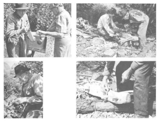
PLATES 74-77 With Mrs. Barnes's and Stan's help, Mr. Barnes selects a small drill and drills two holes—one on the inside end of each bow (*Plate 75*). He then saws off the ends of the bows and, using the scrap, whittles out two hickory pegs (*Plate 76*) and slides them into place (*Plate 77*). These "keys" keep the bows from sliding out.
