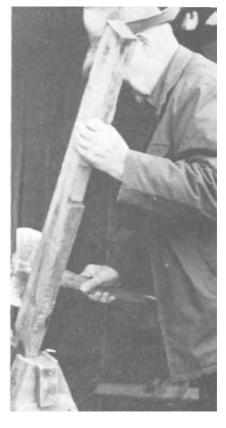
PLATE 171 When the braces for the pedal are in place beside the frame, Greg Strickland drills a hole through both with a brace and bit.
