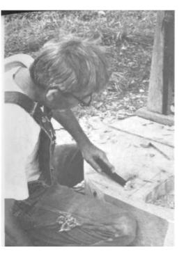
PLATE 143 In the second bucket, Sam finds a piece of wire sticking out of the middle of the wood. Here he tries to ease it out without dulling the edge of his chisel.
