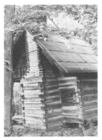
PLATE 372 A beautiful stick-and-mud chimney on a cabin near Brasstown, North Carolina. Note also the gable of hand-split shingles and the wooden shutter with wooden hinges covering the window. Such shutters were used in place of glass, which was not available at the time.
