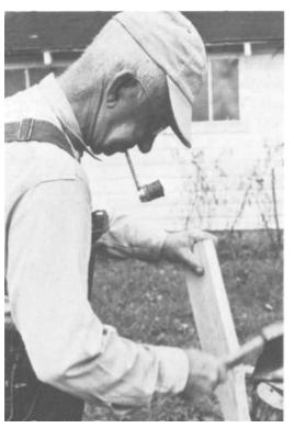
PLATES 323-324 Here he works on the two paddles that are needed. In *Plate 323*, with a drawknife, he shapes in the handle for the stirring paddle. In *Plate 324*, he hews out the handle for the battling stick. The handle will be smoothed as in *Plate 323*. The blade of stirring paddle will be tapered and shaped to fit the bottom of the pot.
