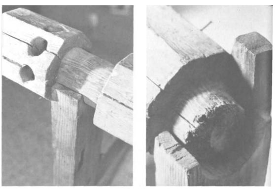
PLATES 270-271 Details of the two ends of the beam in place in the loom frame.
