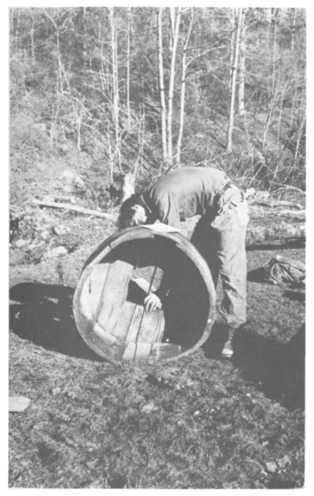
PLATE 167 Ken Kistner measures the wooden housing that fits over the top of the runner rock. Corn to be ground is poured in a hopper which fits in the central hole visible at Ken's left hand.
