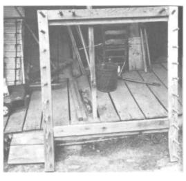
PLATE 294 Minnie Buchanan's handmade warping frame—a little different, but it works on the same principle as Mrs. Brown's.
