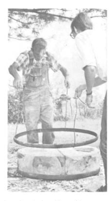
PLATES 147-148 The hoops are then carried to the wheel, red-hot, with hooks, eased over the top, and pounded into place with hammers. Often the hoops are so hot they set the wood afire.
