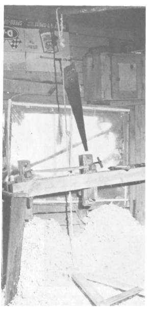
PLATE 181 Of special note are the two end pieces that hold the stock being turned. Rather than being mounted permanently on the vertical support beams, as on Minyard's lathe, these are cross-shaped pieces that slide back and forth between two horizontal beams (as shown here and in *Plate 180*) so that stock of varying lengths can be worked. The stock is held on either end by a metal spike driven through each cross-shaped end piece.
