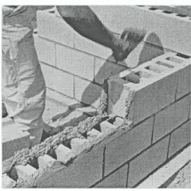
After laying a block foundation, waterproof it with mortar and tar just as poured concrete walls are. In northern climates, the walls should also be insulated, and this can be done in two ways. Either apply rigid foam to the outside of the wall or pour loose fill vermiculite insulation down the block cavities.
