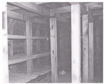
The plywood can be supported very well by rafters supported by 4x4 posts. You will be boxing the form in on top.
